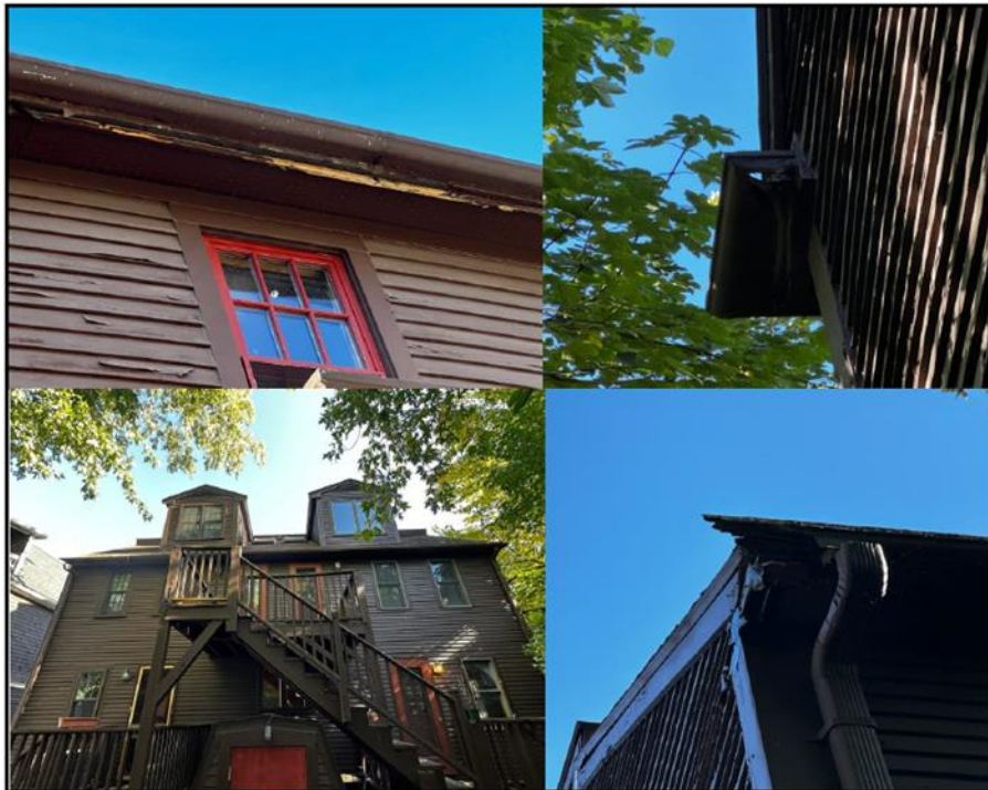
Above: Photos of existing gutter rot at 78 Sycamore St
